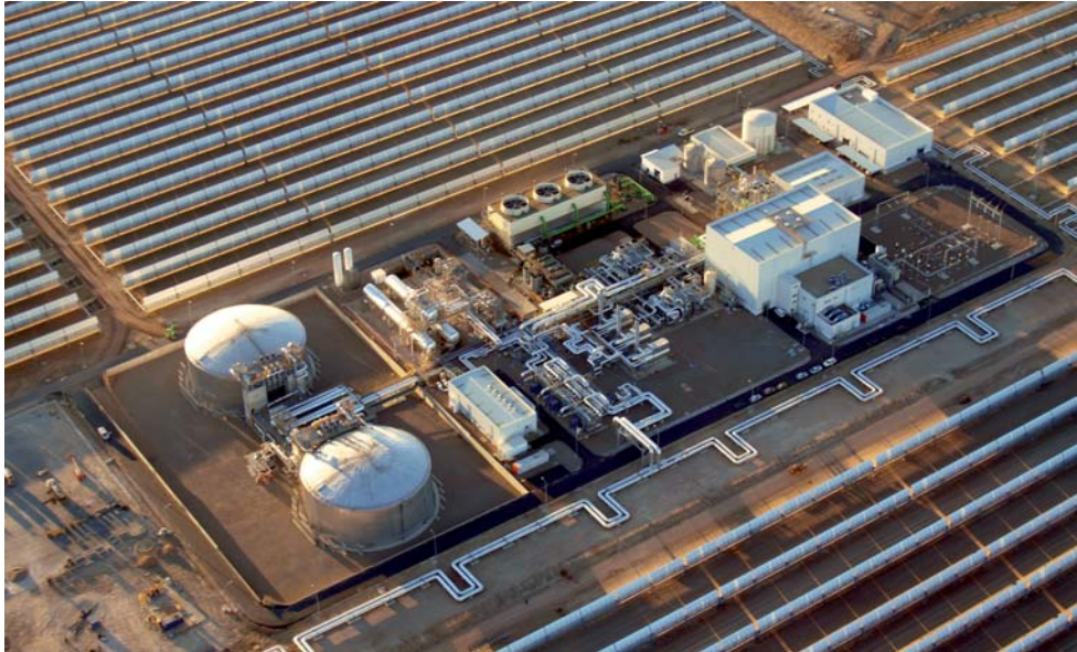
Figure 8. BOP and storage system of the power plant La Florida in Badajoz. Owned by Renovables SAMCA.
